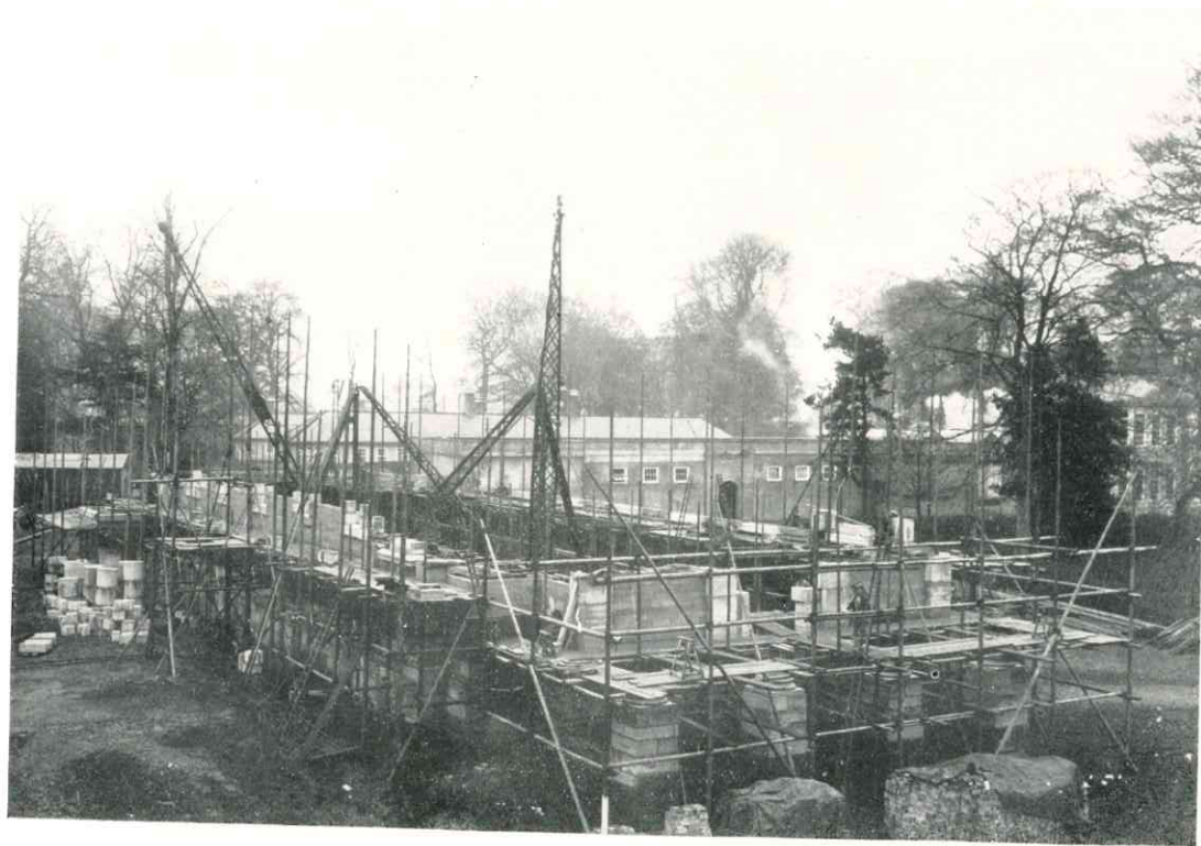
THE CHAPEL—DECEMBER 1ST, 1927.
